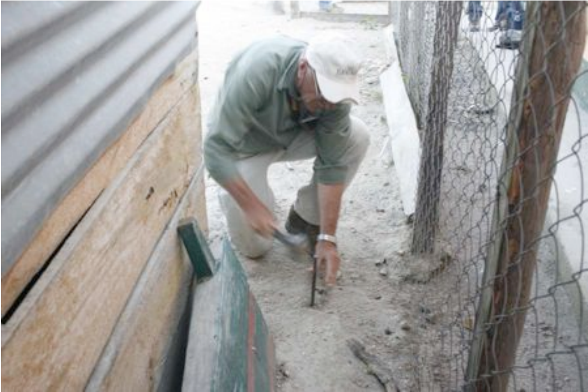
Figure 11 Field Density Test
