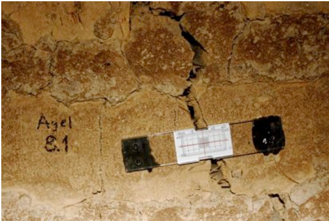
Figure 6b Crack Gauge
