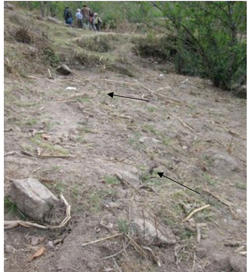
Figure 9d Arrows Show Part of a Fracture that Is 400 Meters Long
