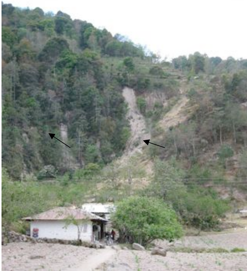
Figure 9c Escarpment (left arrow) and Recent Landslide (right arrow)
